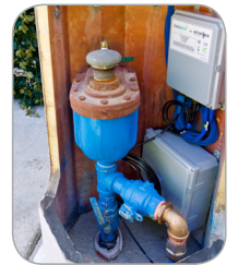
Permanent acoustic sensors installed in chambers are monitoring 4 miles of the water main pipeline installed under Las Vegas Boulevard.
