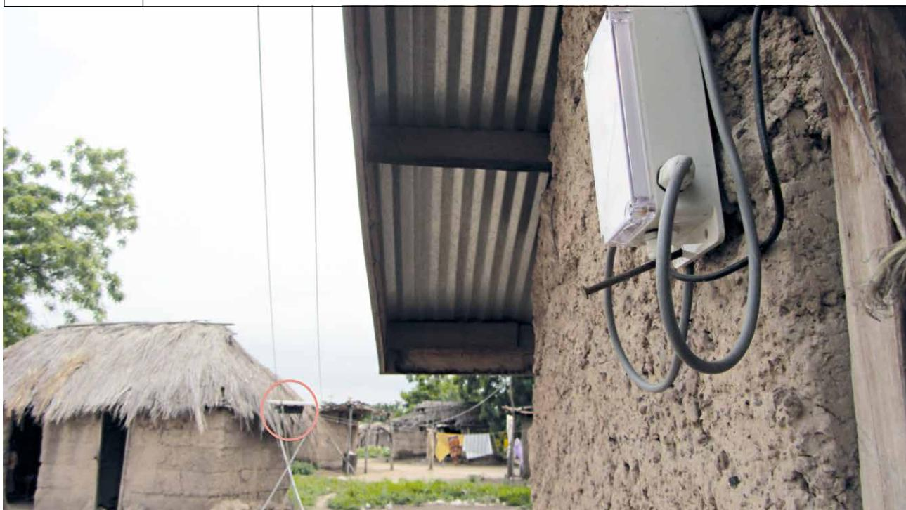
Grid solar panel and battery in the background communicate with the household meter shown in the foreground via ZigBee.
