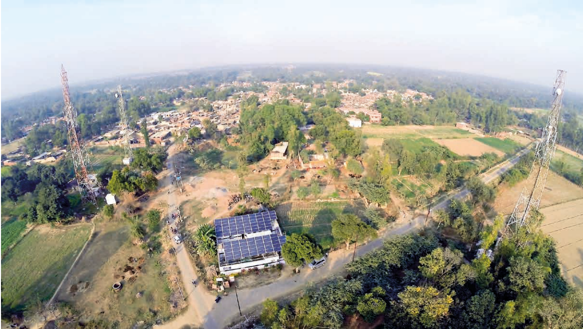
AN AERIAL SNAPSHOT OF A SOLAR POWER PLANT WITH VARIOUS LOADS (SOURCE: OMC POWER)
