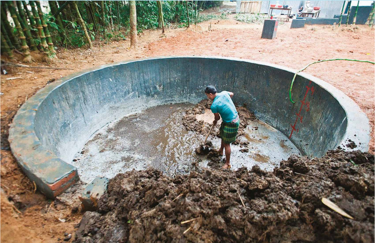
Digester under construction
