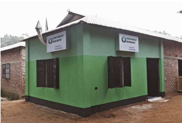
Completed shed at Site 2
