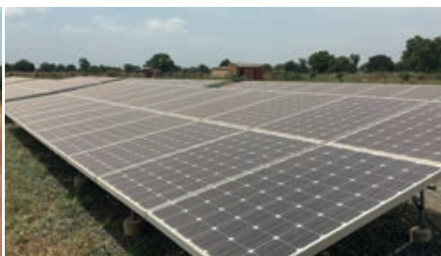
The mini-grid of Bancoumana is one of Access's newest sites. The mini-grid is powered by 144 solar panels and a battery back-up.
