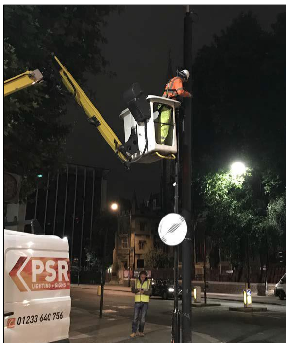
Figure 4: Night-time installation of CCS Metnet nodes
