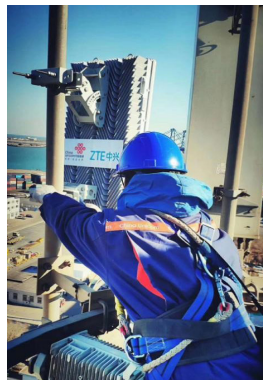
▲ 5G Base Station Installation
