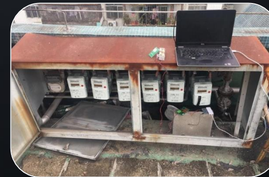
Meter on top of building (with metal cabinet) Path loss: 157.6dB
