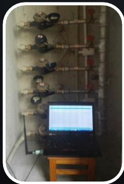
Meter in the wall Path loss: 152.3dB
