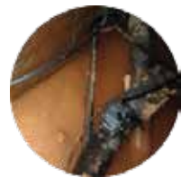
NB-IoT Based Underground Power Cable Temperature Monitoring
