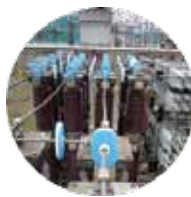
UHV Equipment On-line Diagnosing
