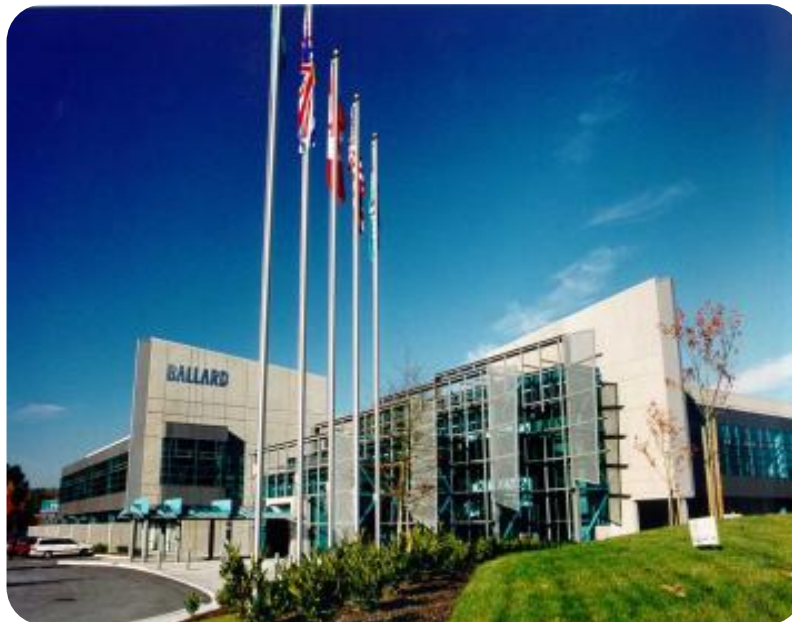
Ballard headquarters facility – Burnaby, BC, Canada
