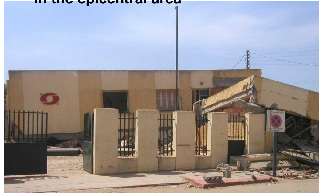
Collapse of the Central Office Building in the epicentral area
