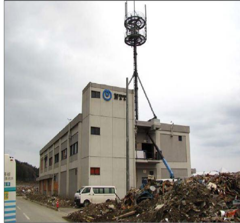
Central Office Building damaged by Tsunami
