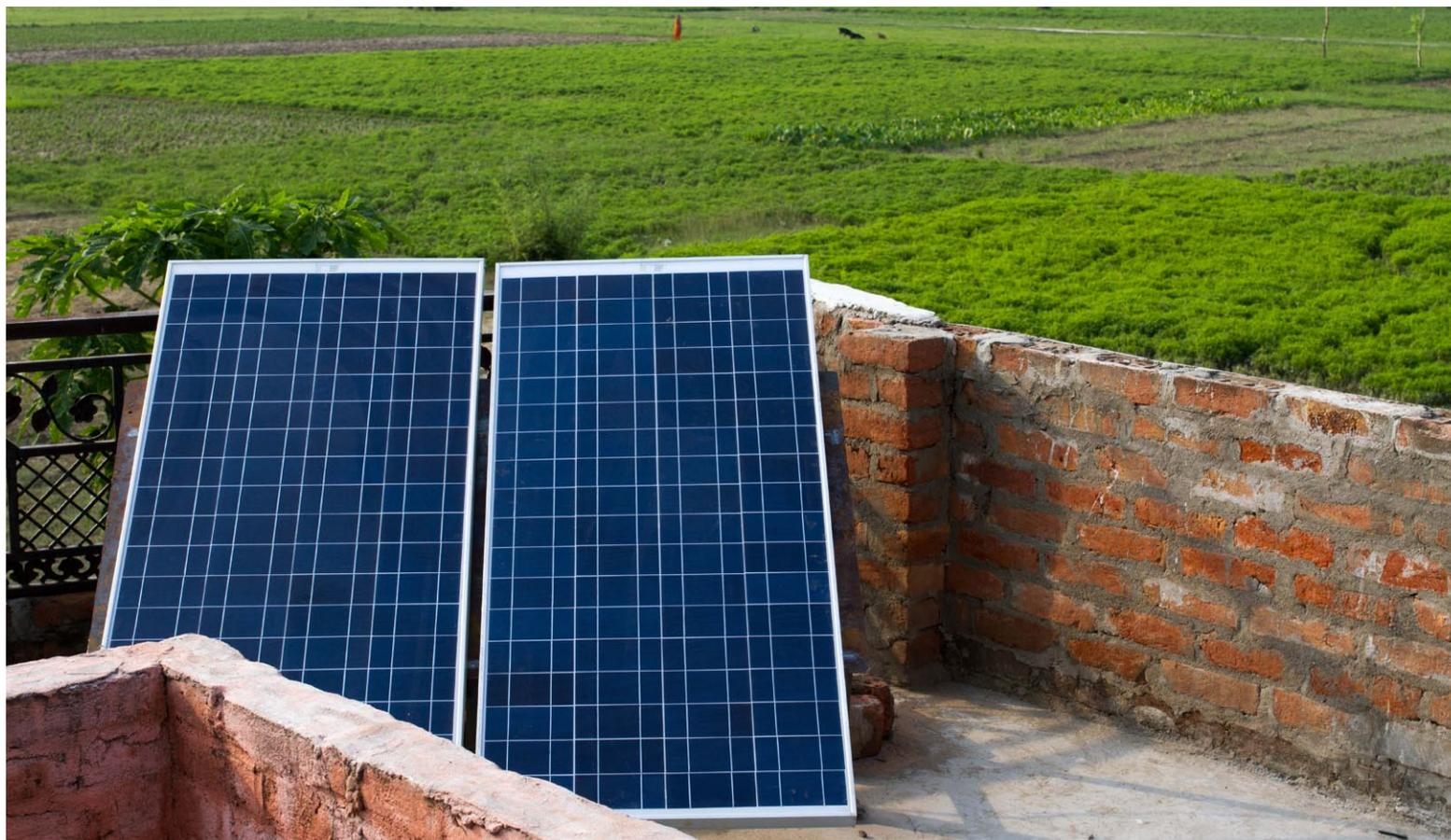
Solar Panels (240W) installed by Mera Gao Power for a microgrid deployment in the Sitapur district - Uttar Pradesh, India.
