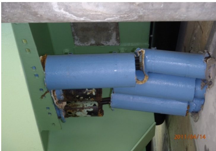
Damage of cable conduit installed under bridge
