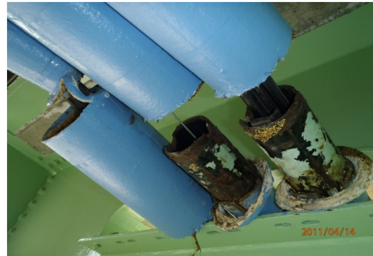
Damage of cable conduit installed under bridge
