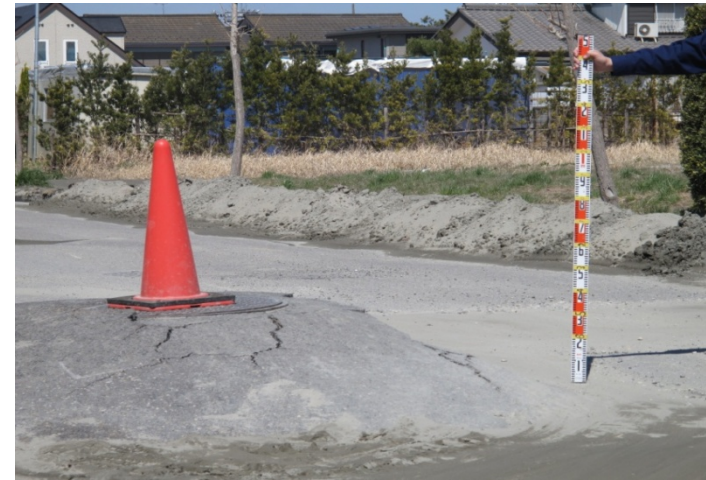
(b) Surfacing of NTT's manhole by liquefaction
