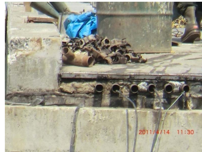
(b) Equipment damaged by falling bridge
