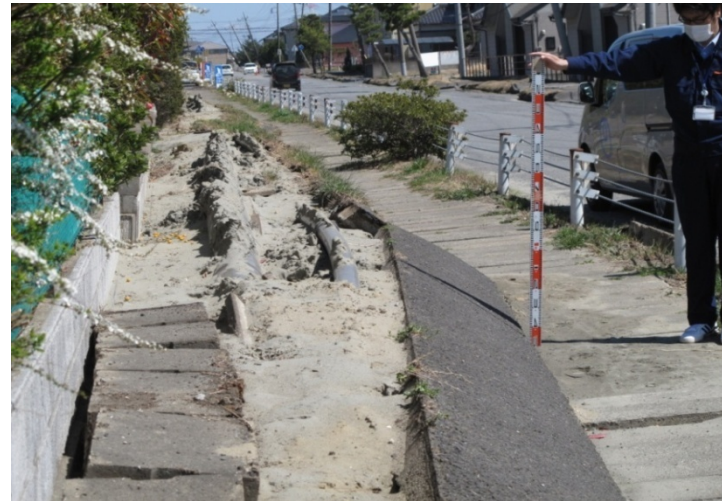
(b) Surfacing drainage tube (about 0.4m)
