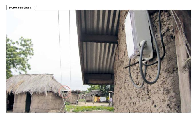
Grid solar panel and battery in the background communicate with the household meter shown in the foreground via ZigBee.
