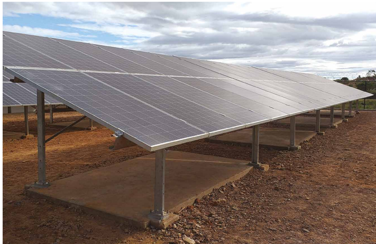
Picture 1: Solar array for the mini-grid in Betsiaka
