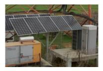
companies. This solar solution has been implemented at more than 1200 sites with installed capacity of approximately 6 MW and generates approximately 8 million units of energy on an annualized basis. The project aims at reducing DG run time from 20 hrs to 5 hrs a day, thus accruing a 60% diesel saving at sites and will thus reduce CO2 emissions by approximately 21,000 MT per year.
