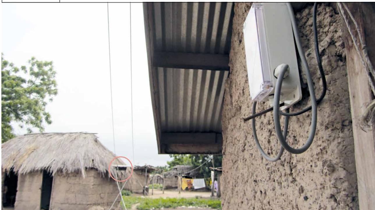
Grid solar panel and battery in the background communicate with the household meter shown in the foreground via ZigBee.
