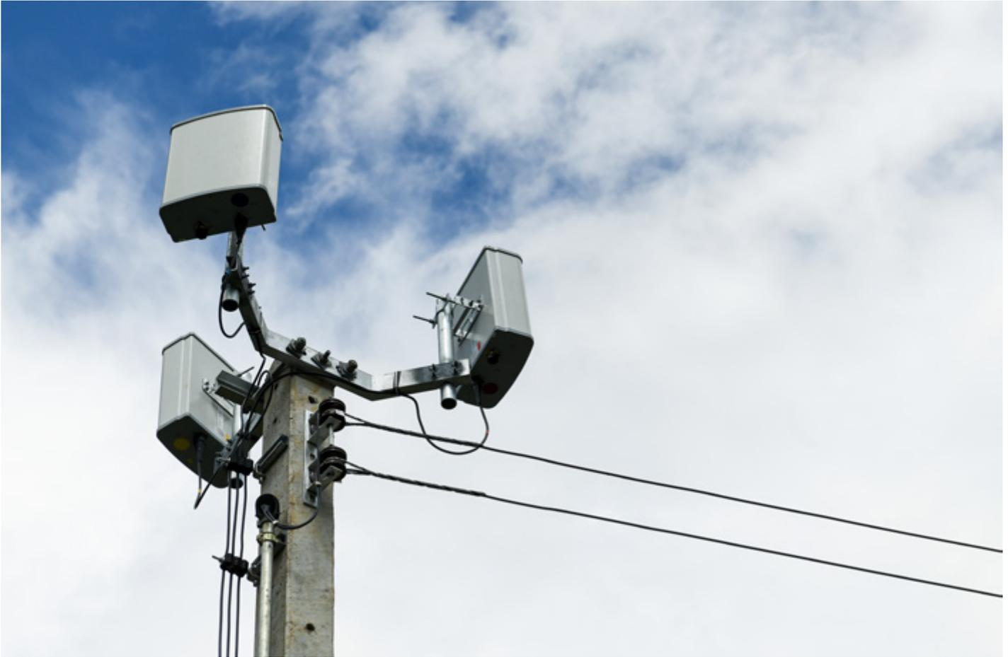
The equipment used for 5G mmWave transmission and reception is smaller than the equipment used for lower frequencies (for example those used for 2G, 3G or 4G). 5G mmWave antennas support beamforming to direct the radio signal to a desired area. Conventional antennas provide coverage that
