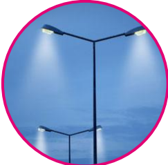
Smart Street Lighting
