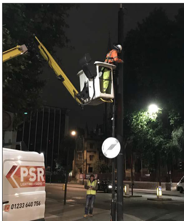
Figure 4: Night-time installation of CCS Metnet nodes
