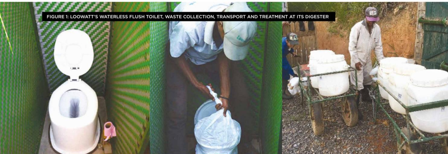
FIGURE 1: LOOWATT'S WATERLESS FLUSH TOILET, WASTE COLLECTION, TRANSPORT AND TREATMENT AT ITS DIGESTER
